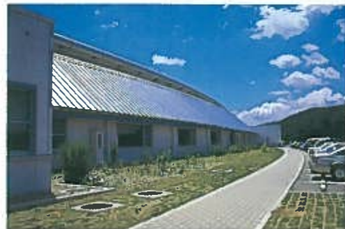
▲The exterior of the Storage Ring Building. From outermost to innermost, the building consists of a corridor, laboratories, experimental hall, and the storage ring (overall length:1,436m).
