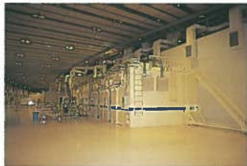
▲An experimental hall inside the Storage Ring Building.
